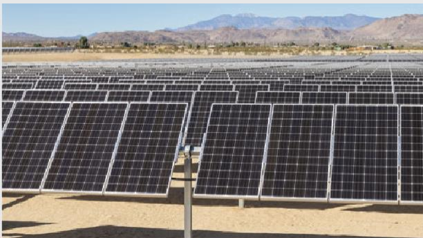
FIGURE 13: The Topaz Solar Farm in San Luis Obispo County is a 550-megawatt photovoltaic power station, one of the world's largest solar farms.
